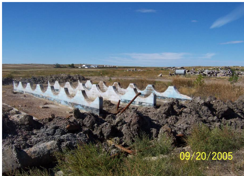
Process Area of the Former Flying J Refinery
