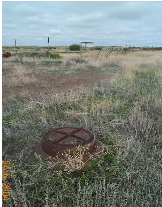
Part of the Refinery wastewater system
