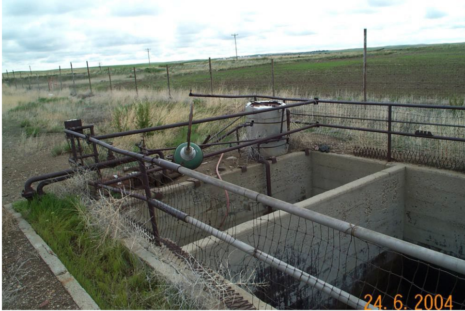
Old API Separator
